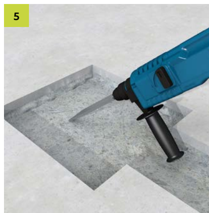
5 If necessary, carry out minor finishing work by hand.
