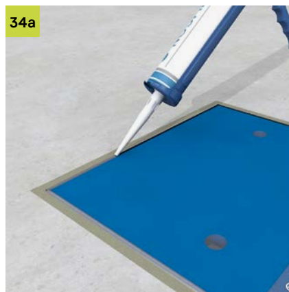
34a To prevent water or dirt from entering the cassette, apply sealant to the joint between the PCX cover and the edge of the cassette.
