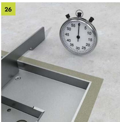
26 Curing times of the potting compound as well as measures to avoid stress cracks, if applicable, can be found in the respective data sheet.
