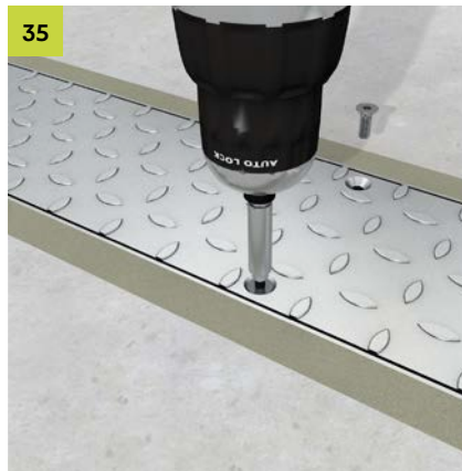
Screw the trunking cover to the trunking tray using the screws supplied. Screw types: UKS M6x16 countersunk screw (ISO 10642).
