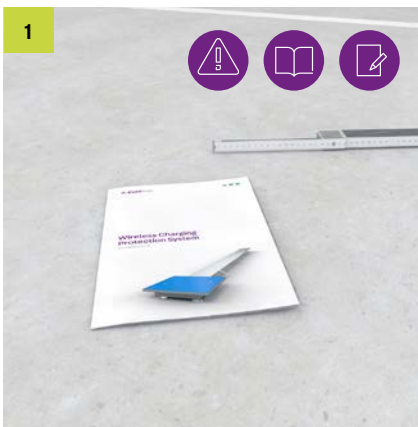
1 Observe floor conditions on site.
