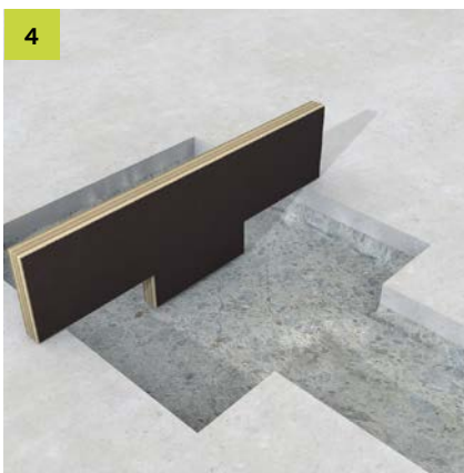
4 Check the quality of the milling. (Depth tester on request)
