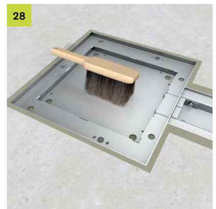
28 Before inserting the loading pad, check for contamination and clean the system if necessary. The channel and cassette must be free of dirt/foreign objects.
