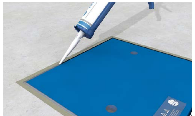
To prevent water or dirt from entering the cassette, apply sealing compound to the joint between the PCX cover and the edge of the cassette.
